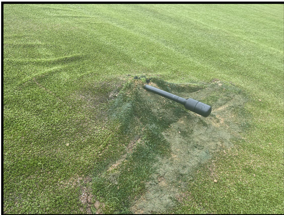
Photograph 2: View of damaged pressure relief vent on west side of Area 1-2.
