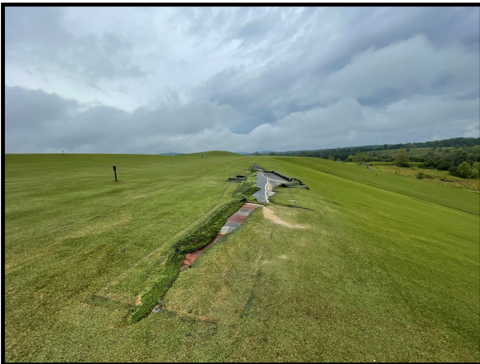
Photograph 4: View of damaged closure turf on east side of Area 1-3.
