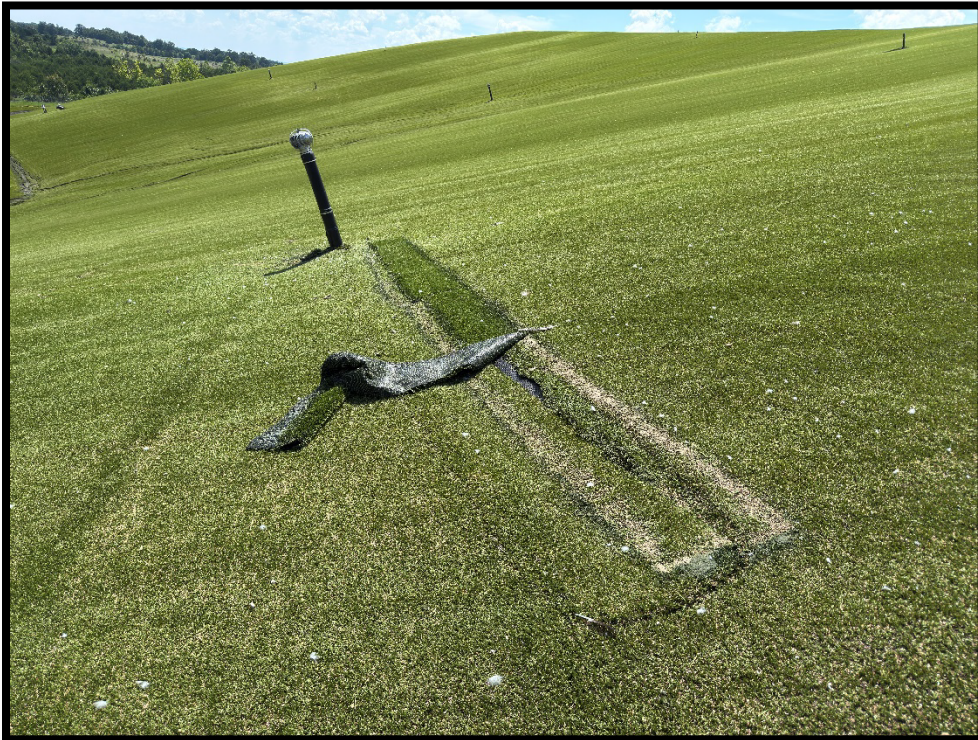
Photograph 3: View of damaged closure turf on the north side of Area 1-2.
